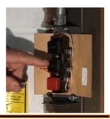
2. Install the new door switch/receiver to the same location on the wall. Install the wires to the 3 switches from which they were removed in Step 1.
